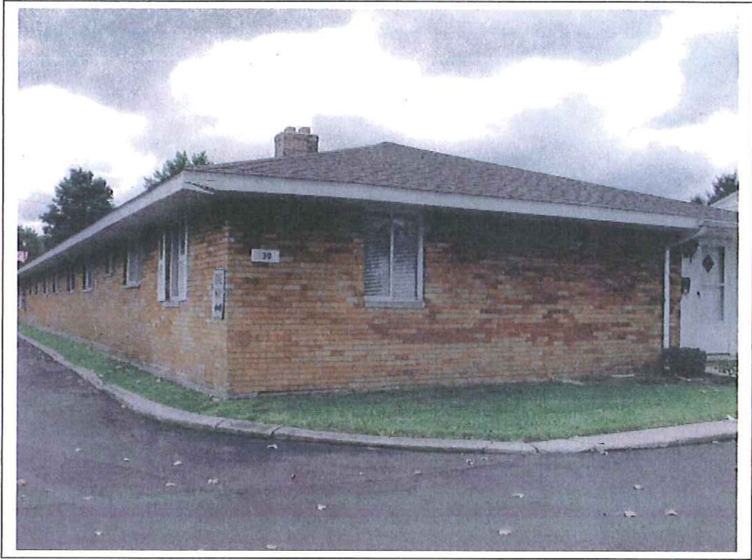
West Side of Third Building
